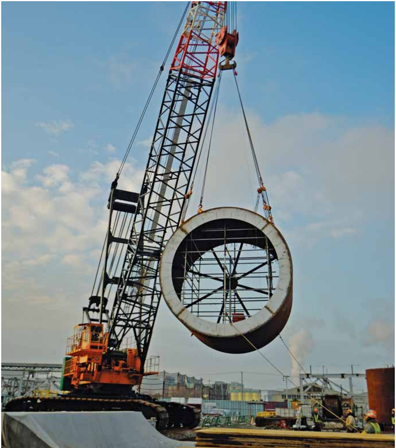
Fast-paced construction at Ishinomaki
