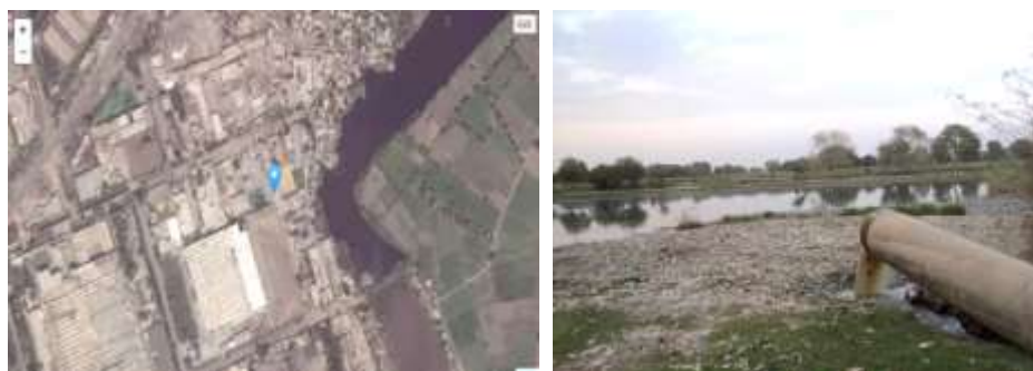
Figure 36.1 The huge dumpsite located at latitude 25.37292 and 68.39581 longitude.
