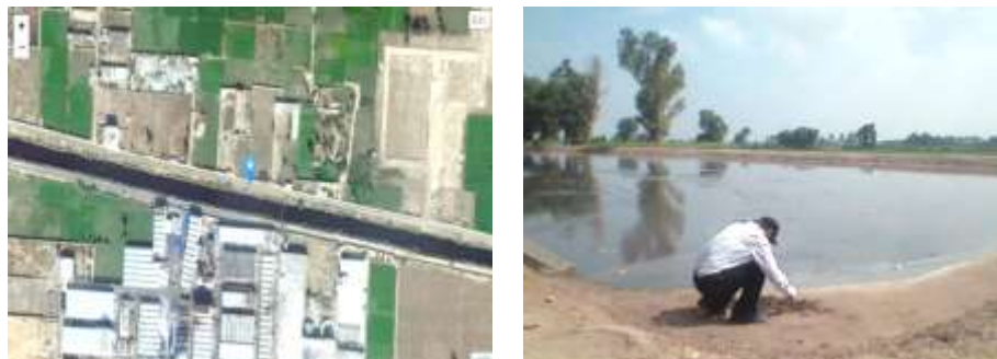
Figure 19.1 The Open pond site was located at latitude 31.39067 and 74.33354 longitude.
