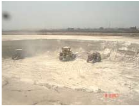
Figure 26.2 Transporting of waste at the site
